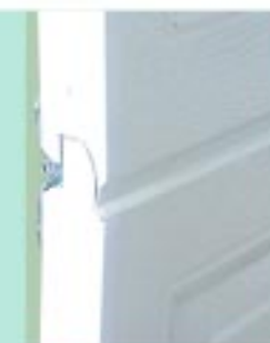
门板拼缝严密、平整 Smooth and tight door panel
