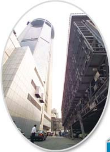
上海新锦江大酒店 PSH-5升降横移式62车位 Shanghai New Jinjiang Hotel PSH-5 Lift-sliding parking system —having 62 parking seats
