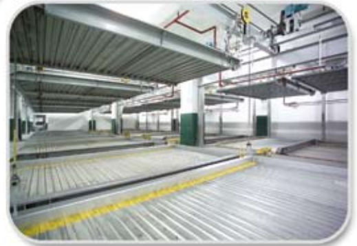
上海音乐广场 二层升降横移 254车位 Shanghai Music Square PSH two-layer Lift-sliding parking system—having 254 parking seats
