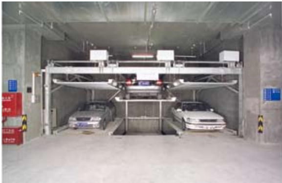
PSH2.3.4.5层升降横移自动化停车设备 (参数表) PSH2.3.4.5Lift-sliding mechanical Parking System
