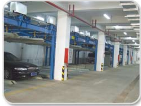
山西国家安全厅 PSH-2升降横移式 76车位 Shanxi Provincial Security Department PSH-2 Lift-sliding parking system—having 76 parking seats
