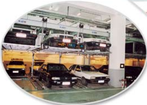
上海二中院 PSH-2升降横移式 215车位 Shanghai Erzhongyuan PSH-2 Lift-sliding parking system—having 215 parking seats
