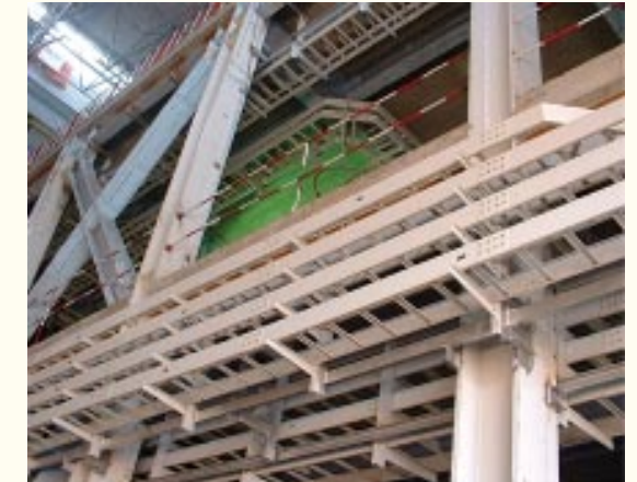
Tangshan Thermal Plant Project, Hebei Province (Cable Tray)
