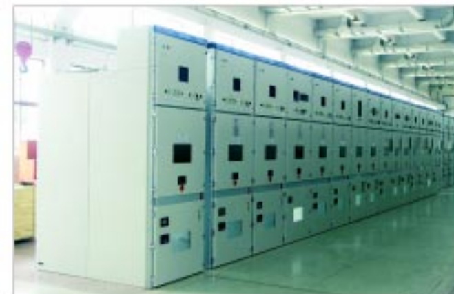
KYN28-12 AC Armored Metal-enclosed Switchgear
