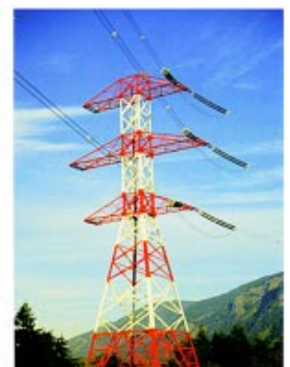
110KV Angle Tower
