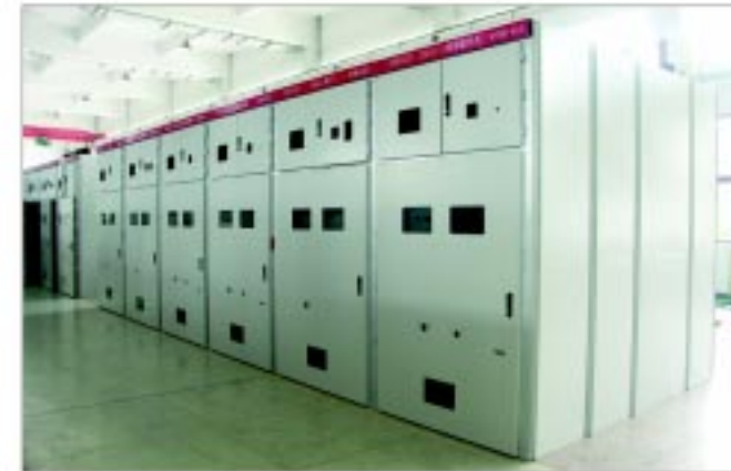
KYN61-40.5 AC Armored Metal-enclosed Switchgear
