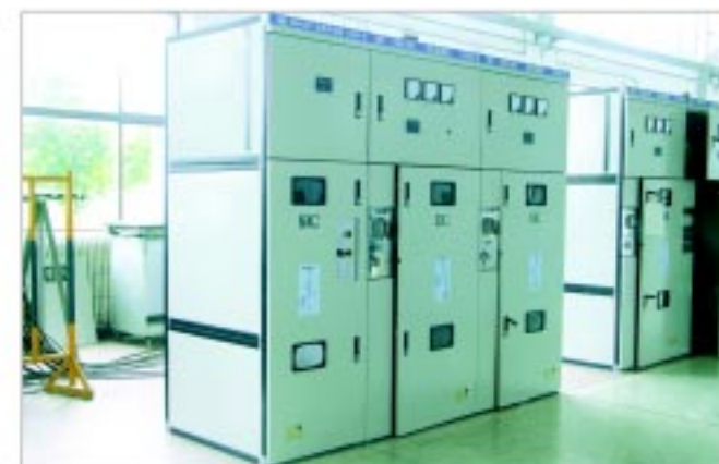
XGN2-10 AC Metal-enclosed Switchgear
