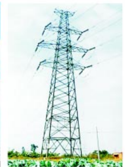
220KV Double-circuit Angle Tower
